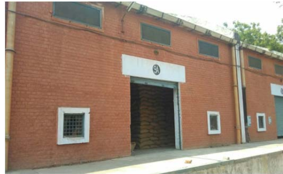
Fig. 1. Grain storage shed kept open for aeration
